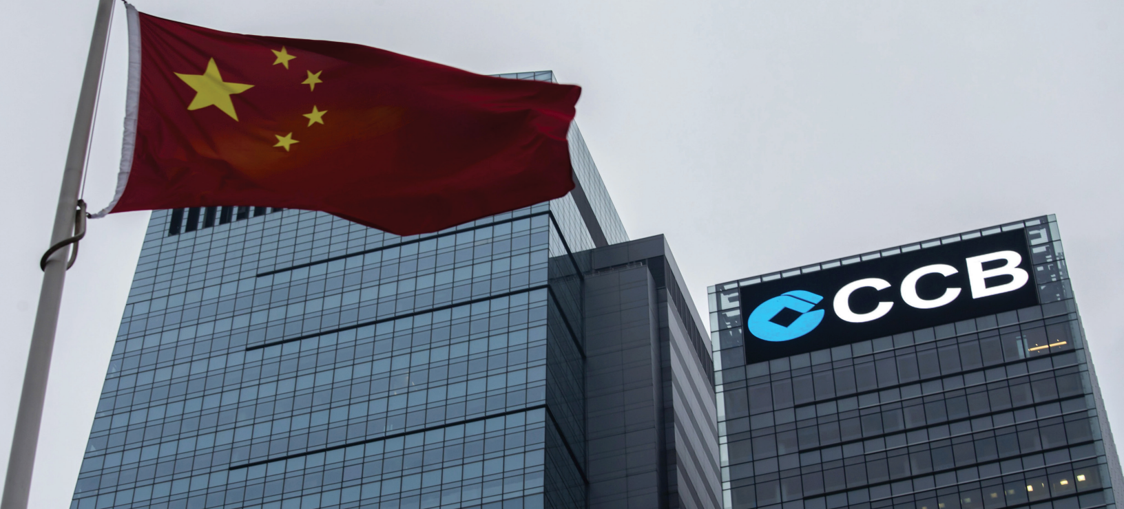
A Chinese national flag flies in front of the China Construction Bank (CCB) Tower at Hong Kong's business Central district in this December 26, 2014 file picture. REUTERS/Tyrone Siu/Files
